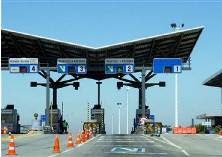
Example of VIA VERDE station interoperable with the Via T
