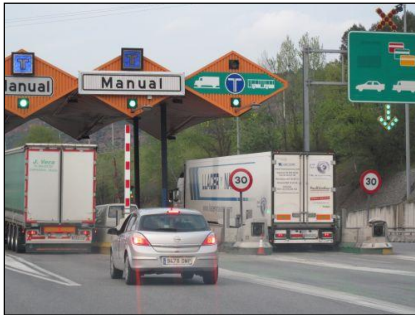
Example of a VIA-T station
